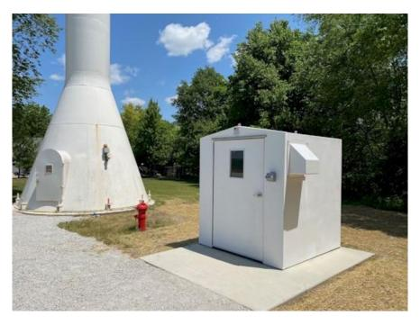
Our chemical treatment building has been installed and is operating. Chlorine treatment previously done inside the water tower base is now being processed in the new building. This will eliminate the corrosive impact of the chlorination process on the water tower base interior. Moving this process out of the water tower was also required prior to beginning the water tower refurbishing project.
